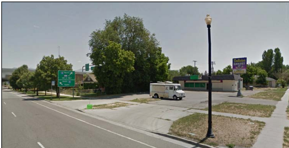
Street View of Properties Proposed for Rezoning at the Southwest corner of the Intersection
